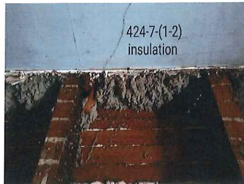
424-7 Insulation Typical interior
